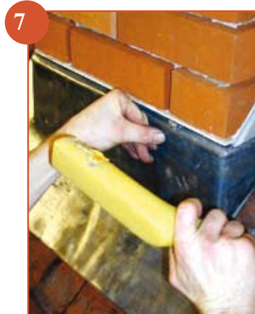
7 The lead is then dressed securely into the flashing channel
