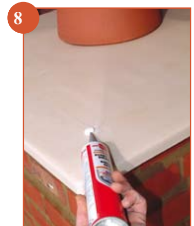
8 The lifting eye plugs must be sealed into the lifting eyes to finish
