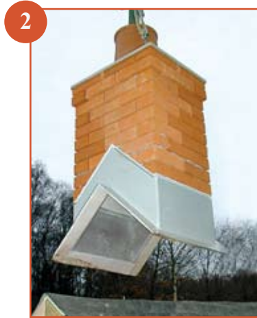
2 Crane into position on the trusses using the lifting eyes and loops supplied
